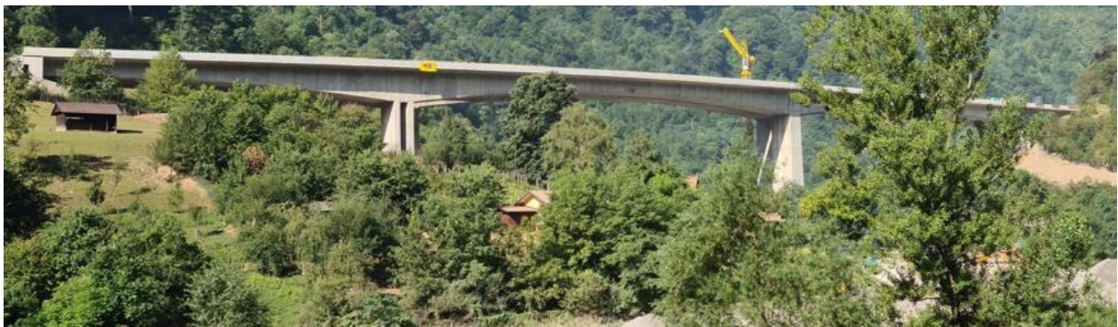
Figure 34. Vranduk 1 left and right bridge
