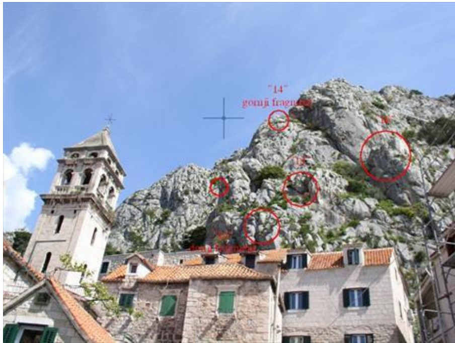
Figure 1.2: Omiš city centre under the danger of potential rock falls
