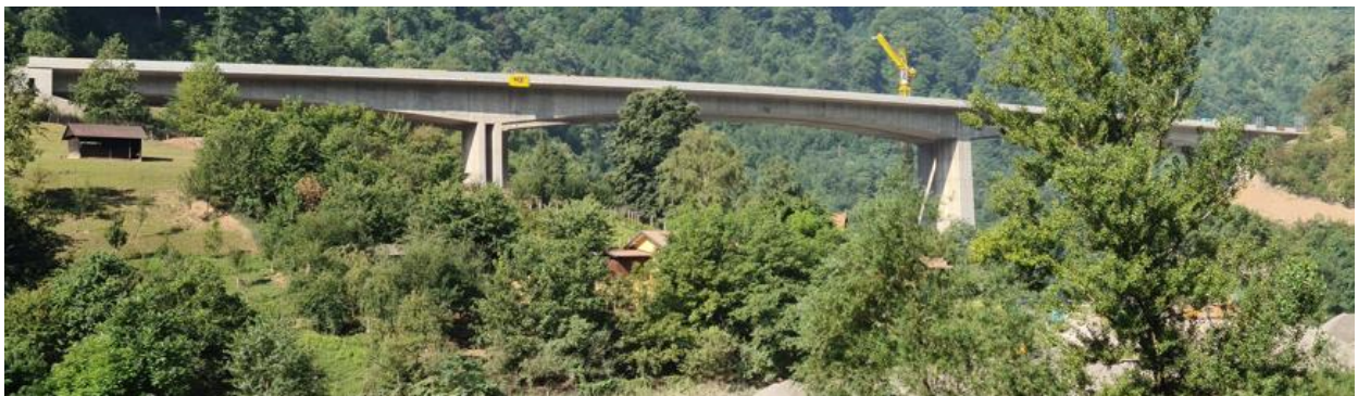
Figure 34. Vranduk 1 left and right bridge
