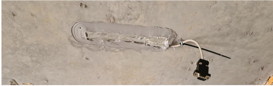
Figure 50. Strain gauge after protection
