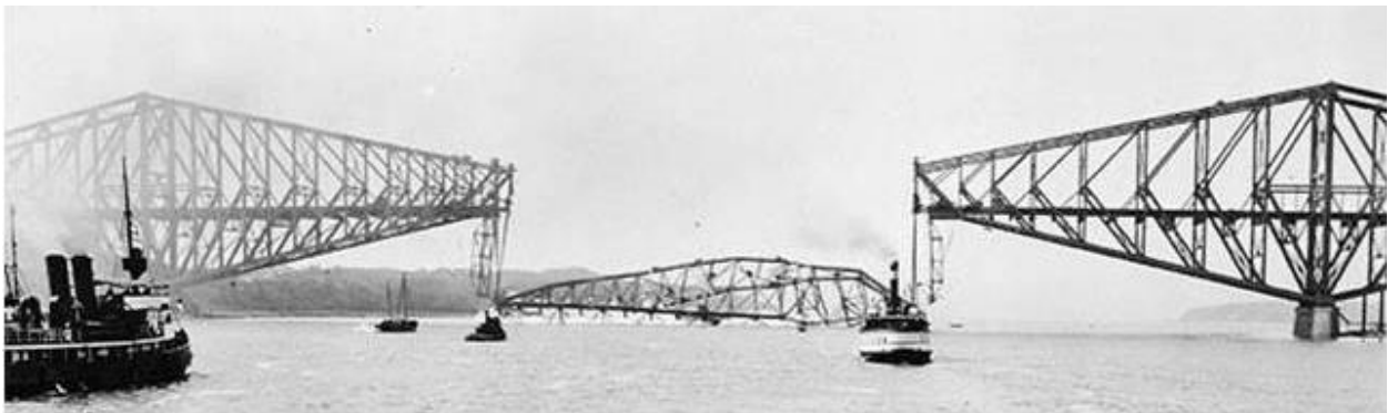
Figure 19. Quebec bridge, collapse of the central segment
