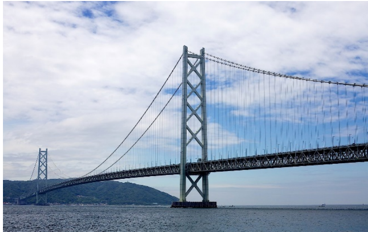
Figure 2: Akashi Kaikyo Bridge in Japan - the longest central bridge span ever built. Photo courtesy of http://broer.no .
