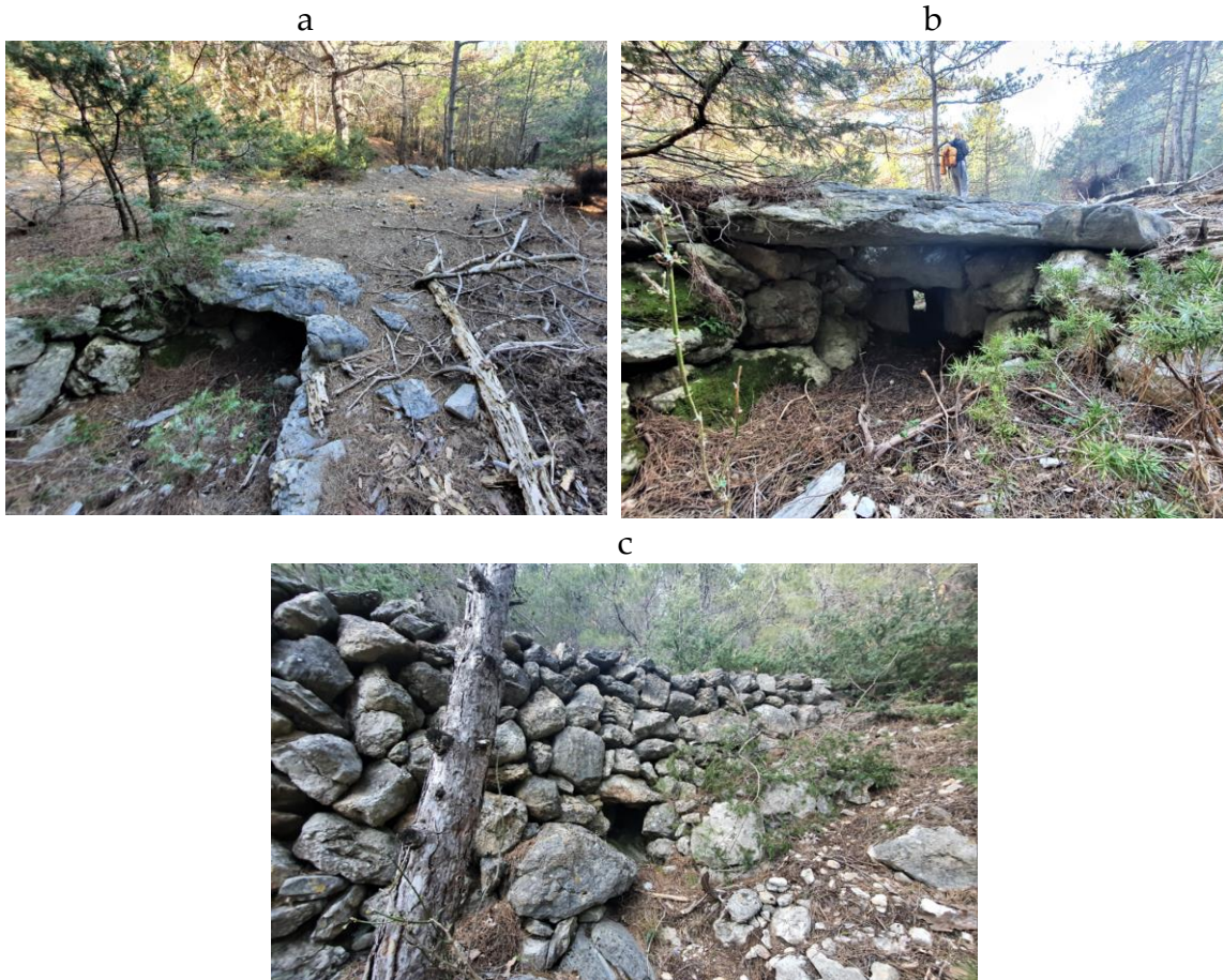
Figure 64. A water conduit below the pathway Germov in Miholašćica (2021)
