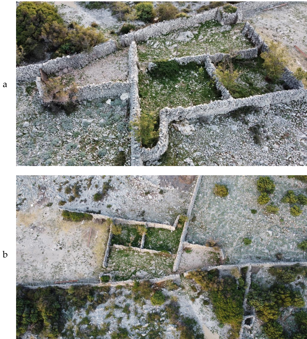
Figure 52. The multicellular sheepfold Mihojski . a) The two upper partitions are currently the only ones in active use. b) The pregrājić is the wider space at the entrance to the mrgar , visible on the left side of the photograph. Two przgari are visible; the left one belongs to the Mihojski sheepfold (2020).
