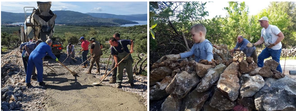
Figure 187. The annual work of the members of the Cres olive growers’ association ‘Ulika’ of concreting the roads to olive groves in order to facilitate agricultural production, but at the expense of the vernacular dry stone architecture (© Franko Fučić)
