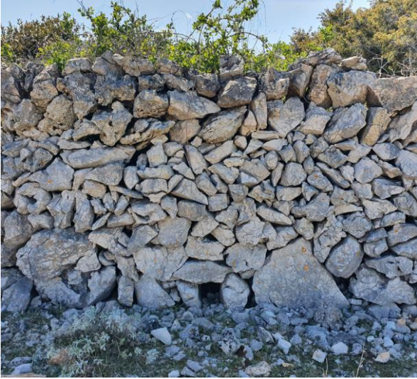
Figure 111. Smout holes ('pasaji za zece') a) close to Loze (2021) and b) in the Osor environs (2021)
