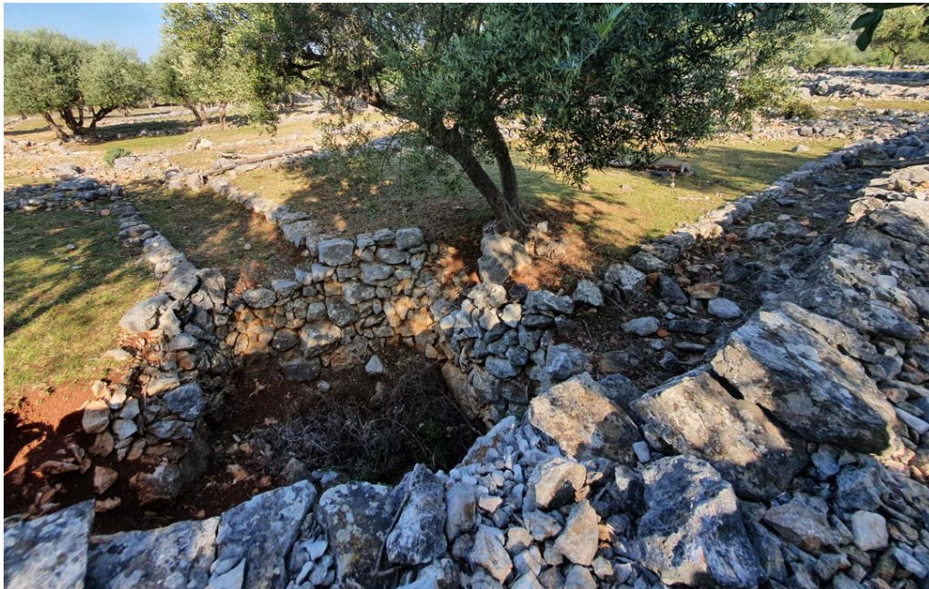
Figure 56. From right to left: a canal entering a dry stone-lined cistern, with stairs below the second canal that funnels the water to the next parcel when the cistern is full (2020).
