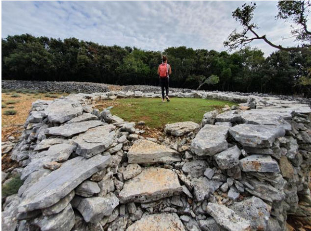
Figure 125. An elevated threshing floor in Veli Tržić: a) a rim covered in stone slabs, with a staircase, b) in the foothills of Osorščica (in the back) (2020)
