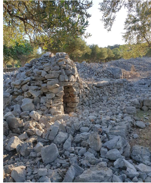
Figure 98. A dry stone hut with a square ground plan and a corbelled roof of stone plates, between the bays of Banja and Kruščica (© Dorijan Lovrečić, 2020)
