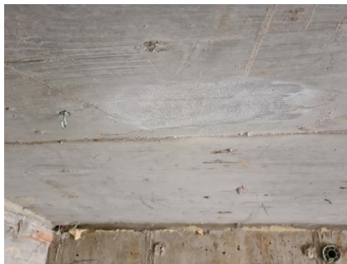
Figure 48. Surface prepared for gauge installation
