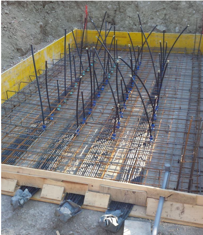
FIGURE A.19: Installation of piezometers.
