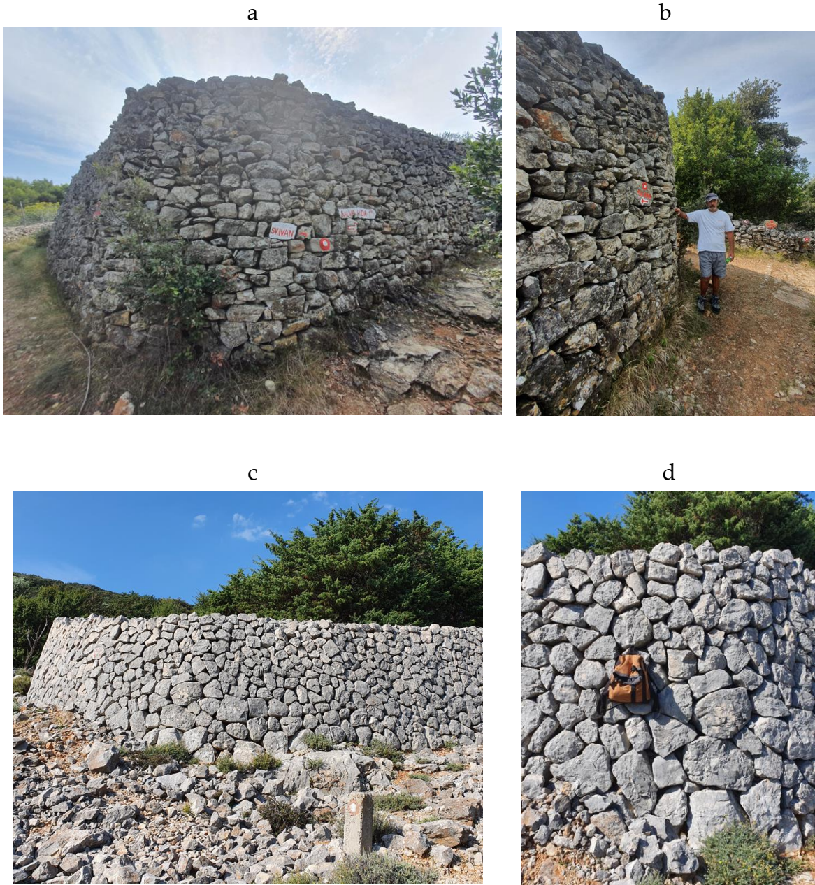
Figure 7. Rare examples of hewn dry stone structures on the Cres and Lošinj islands. These outer walls represent the lower retaining walls a-b) along the pathway from Veli Lošinj to Sveti Ivan (2020) and c-d) Along the gravel road from Cres to Valun (2020)
